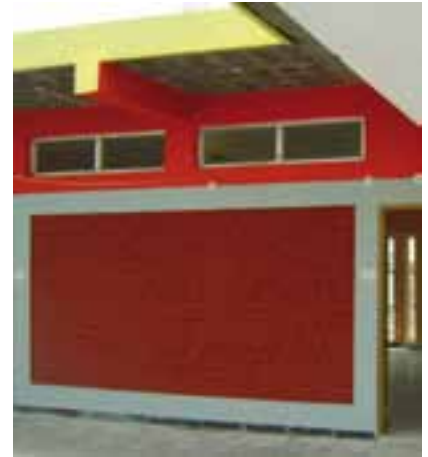
Figure 4 Demonstration of filler slab and unplastered walls in the constructed building
